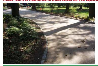
NOTE: A suitable steel, wood, brick, stone or aluminium edging should be provided to ensure a neat edge detail.
